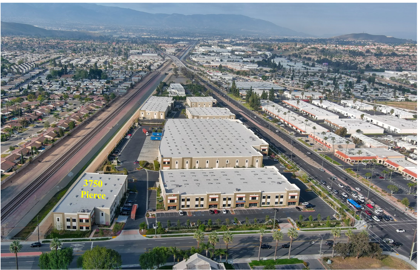
3750 Pierce Street, Riverside CA 92503
